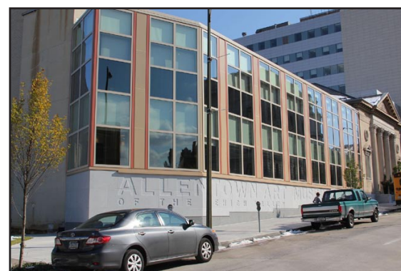
The expanded and renovated building reopened on October 16, 2011
